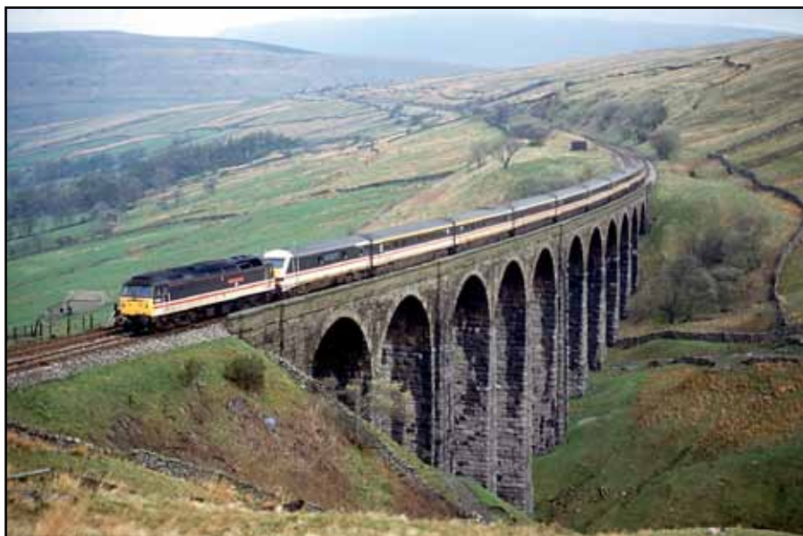
Below: 47973 Derby Evening Telegraph plus Driving Van Trailer, on 1M18 the 07.05 Glasgow-Euston, crossing Arten Gill viaduct in Dentdale; 24/4/1993. Photos: Pete Shaw
